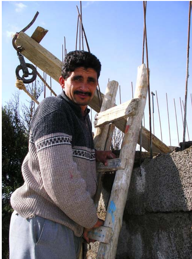
Figure 4: Association President inspecting water tower project
