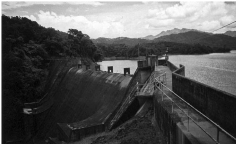
The Lago Guayo dam, a large structure that blocks shrimp and fish migration and causes the upstream decimation of native shrimp and fish populations in Puerto Rico.
